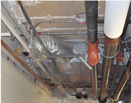
CHILLED WATER PIPING
