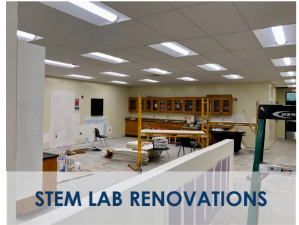
STEM LAB RENOVATIONS
