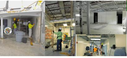
Contractors are keeping busy at Pompano Beach Middle School. The locker rooms have been gutted in preparation for renovations, ductwork is being replaced in multiple buildings, roofing repairs are being made, and all buildings are being repainted.
